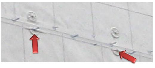
When installing discs adjacent to one another, be careful not to overlap; otherwise, there will be an air passage at the overlap, and the two discs need to be encased in sealant.
